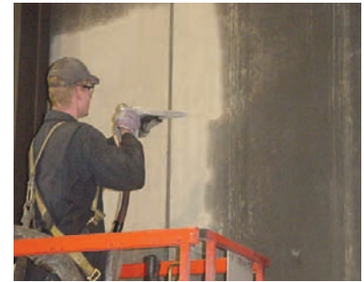
fire damage - soot on concrete
