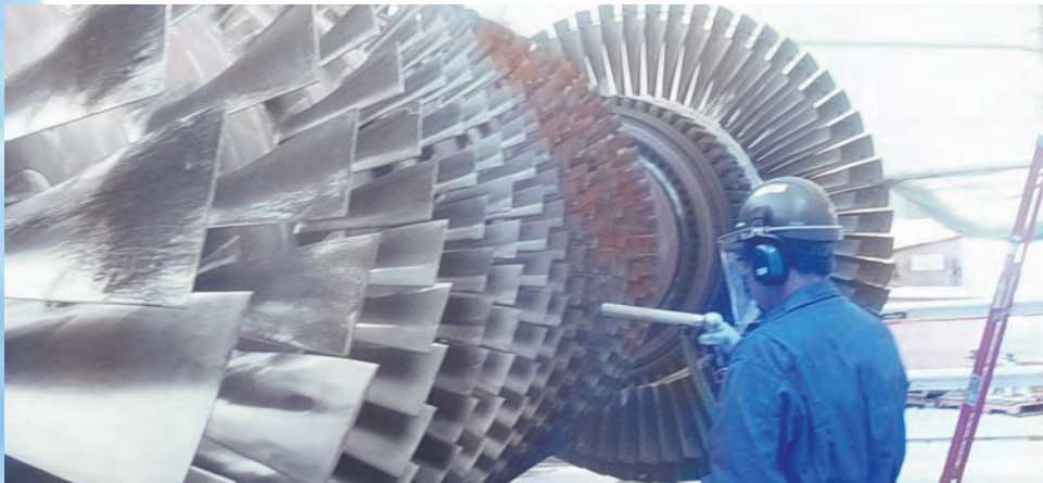
utilities - turbine generator cleaning
